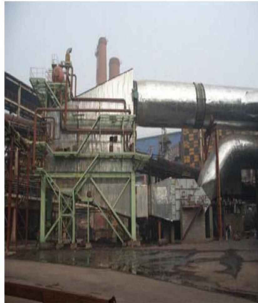
Waste heat recovery power plant for sintering cooler
