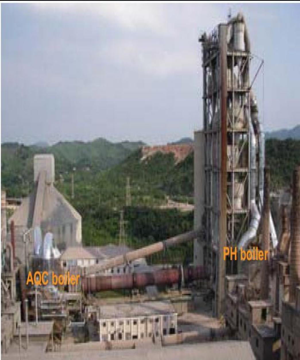
Waste heat recovery power plant for cement plant
